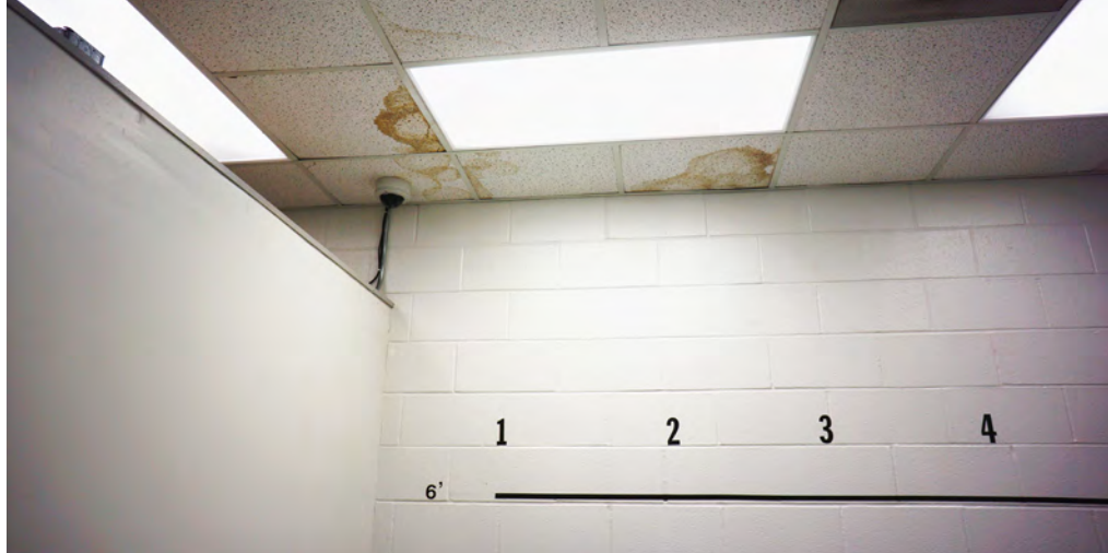
The ceiling in the Police Station’s Lineup Room shows signs of water damage from high humidity and water leaking.
