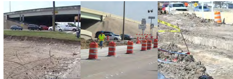
Figure 7.4, Highway 290 Construction Activities
